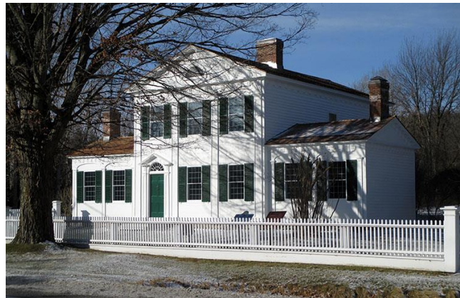
Barnum House, Grafton Ontario Built 1817-1819 by Ellakim Barnum, a United Empire Loyalist originally from Vermont
